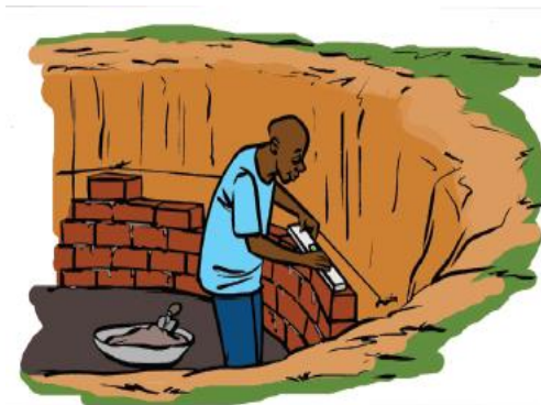
5. Use of spirit level to ensure proper levelling
