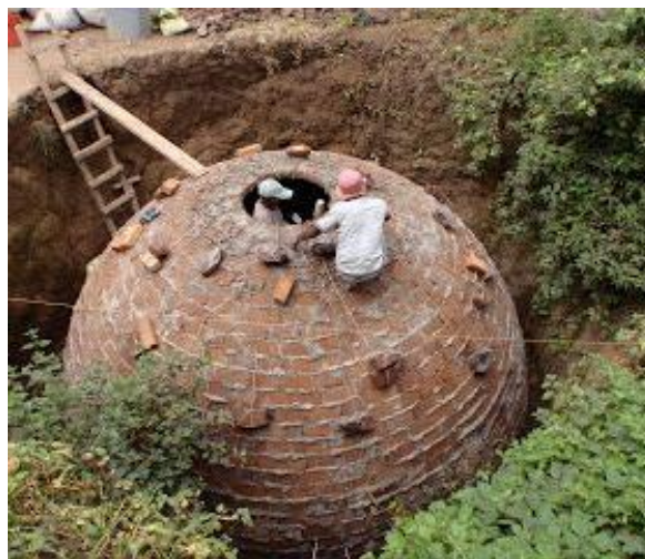
Brick masonry underground tank
