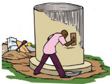
7. Plastering work and water proofing
