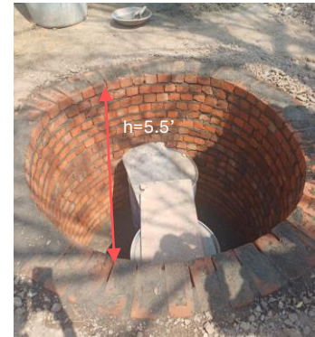
Brick Masonry Underground Storage Tank
