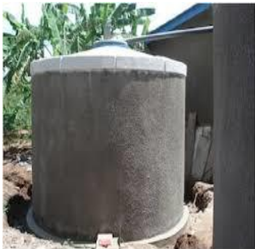
Ferrocement tank- underground
