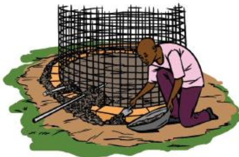
5. Brickwork and installing washout pipes
