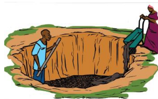
3. Construction of tank foundation
