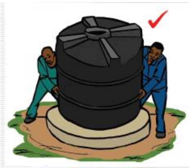
3. Erecting Plastic tank on raised platform
