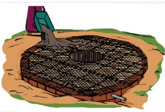
6. Construction of concrete cover
