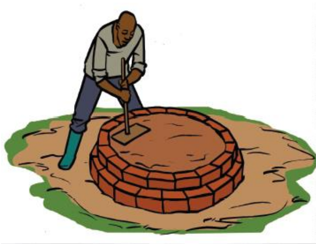
1. Constructing raised platform using bricks and cement
